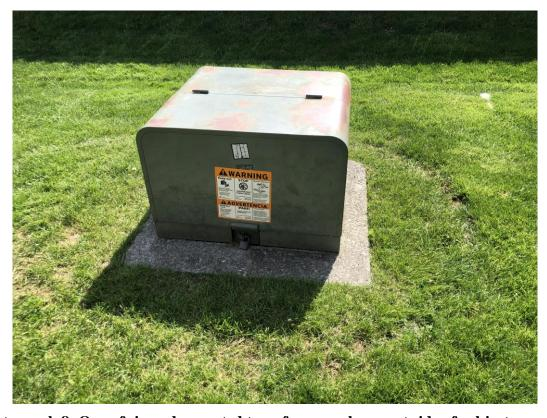
Photograph 8: One of six pad-mounted transformers along east side of subject property
