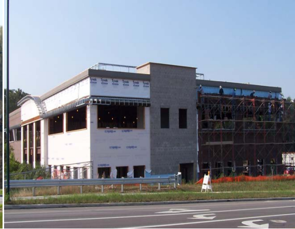
Central Ohio Urology Group Under Construction
