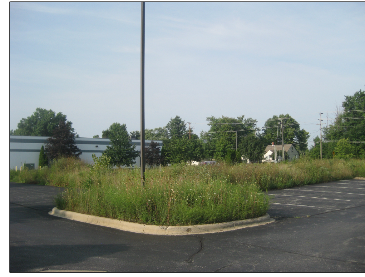
3 VIEW FROM NORTH EAST CORNER
