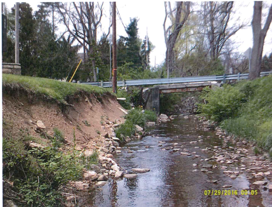
Photograph No. 1 –Looking North/Upstream from South Entrance
