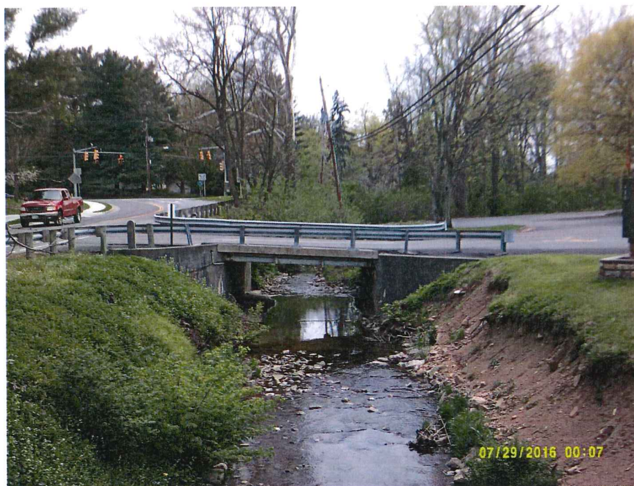
Photograph No. 2 –Looking South/Downstream from North Entrance
