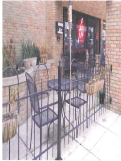
existing railing KTS
