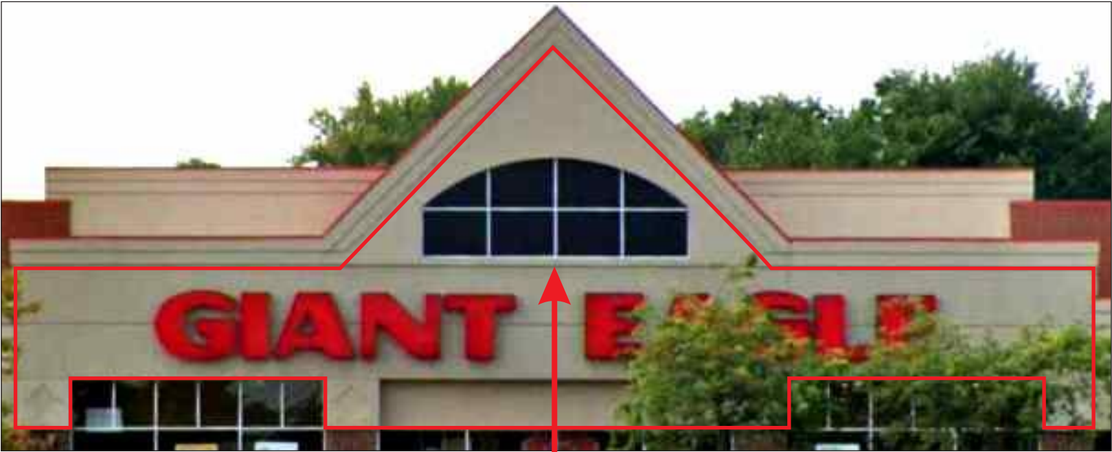
AREA OF REPAIR REPAIR, PATCH, & PAINT AREA (SCRATCH, RESURFACE, & EFIS REPAIR) WHERE EXISTING LETTERS WERE REMOVED. PAINT TO MATCH AREA OUTLINED IN RED.
