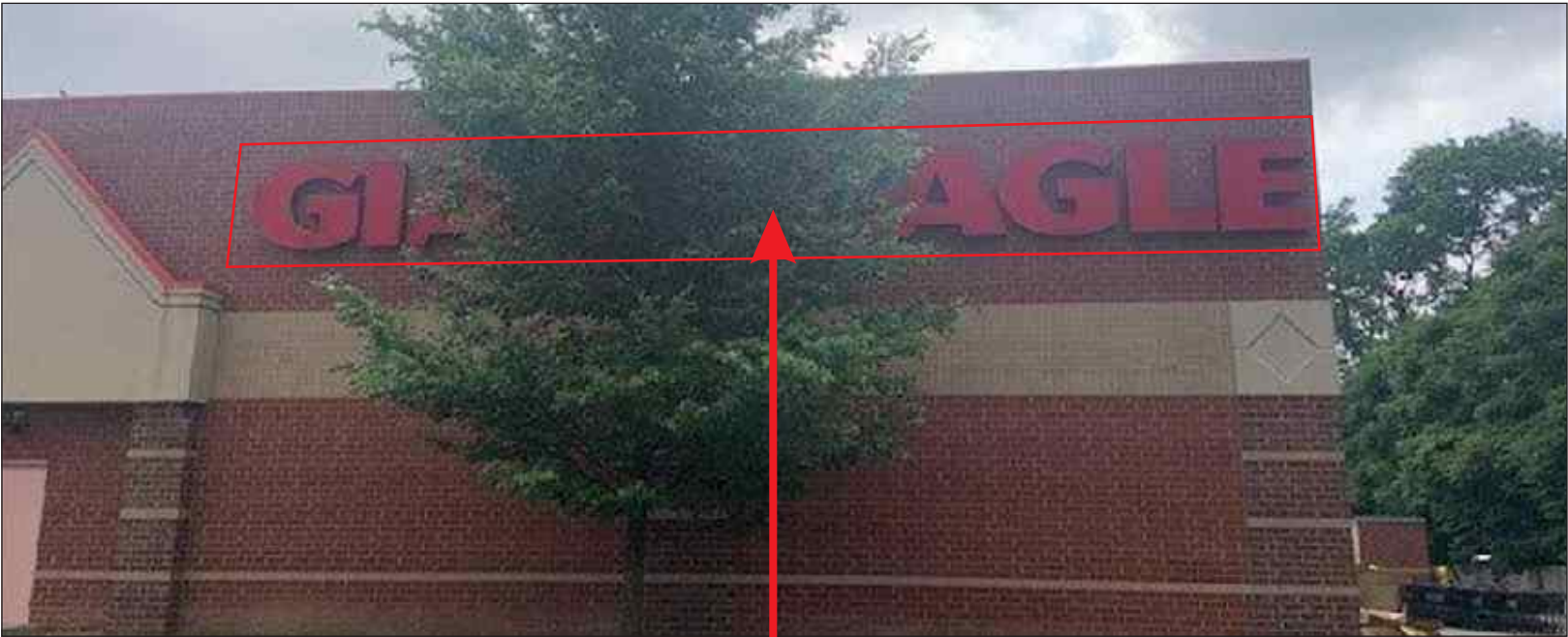
AREA OF REPAIR AFTER REMOVAL OF EXISTING SIGN, HOLES IN BLOCK WALL WILL BE PATCHED WITH MORTAR MIX, COLORED TO MATCH EXISTING BLOCK.
