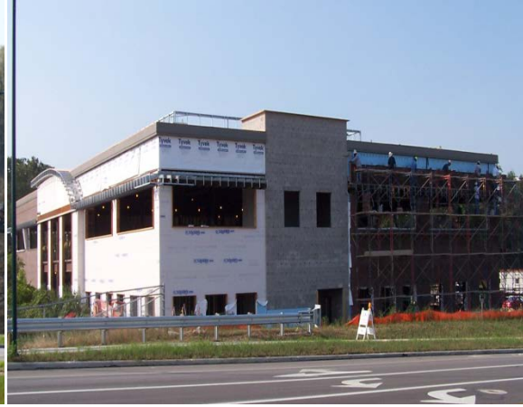
Central Ohio Urology Group Under Construction
