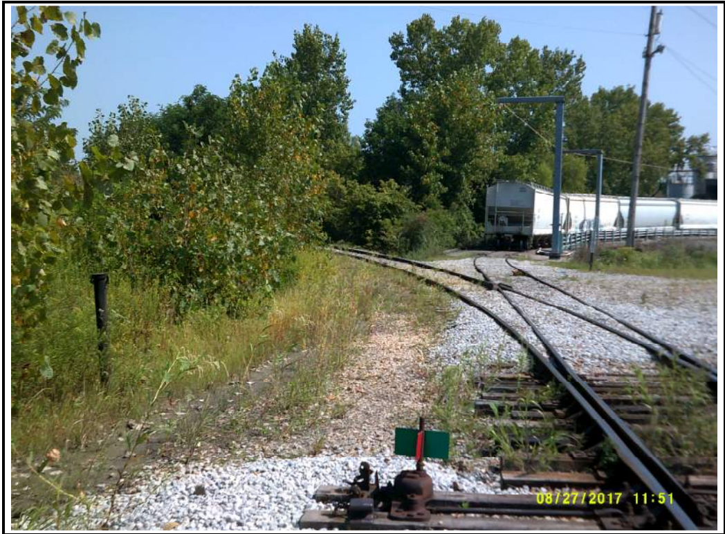
Photograph 19: Rail west toward split.
