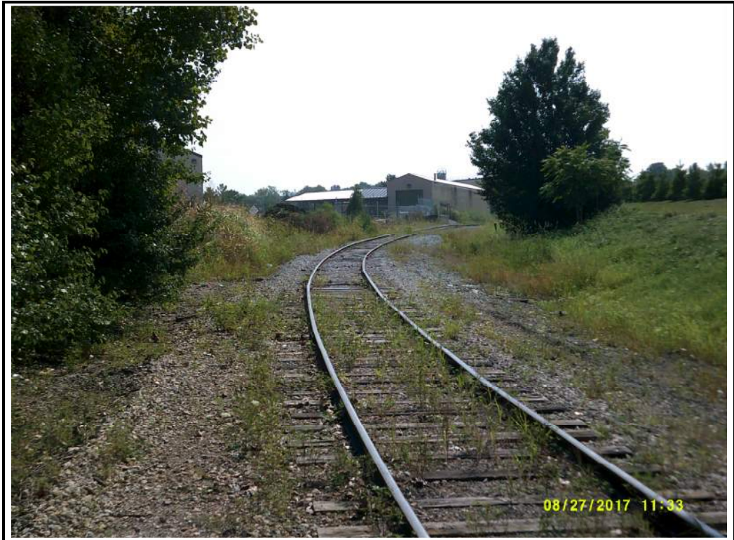
Photograph 7: Rail looking east toward hedge. Geiger Excavating on right.
