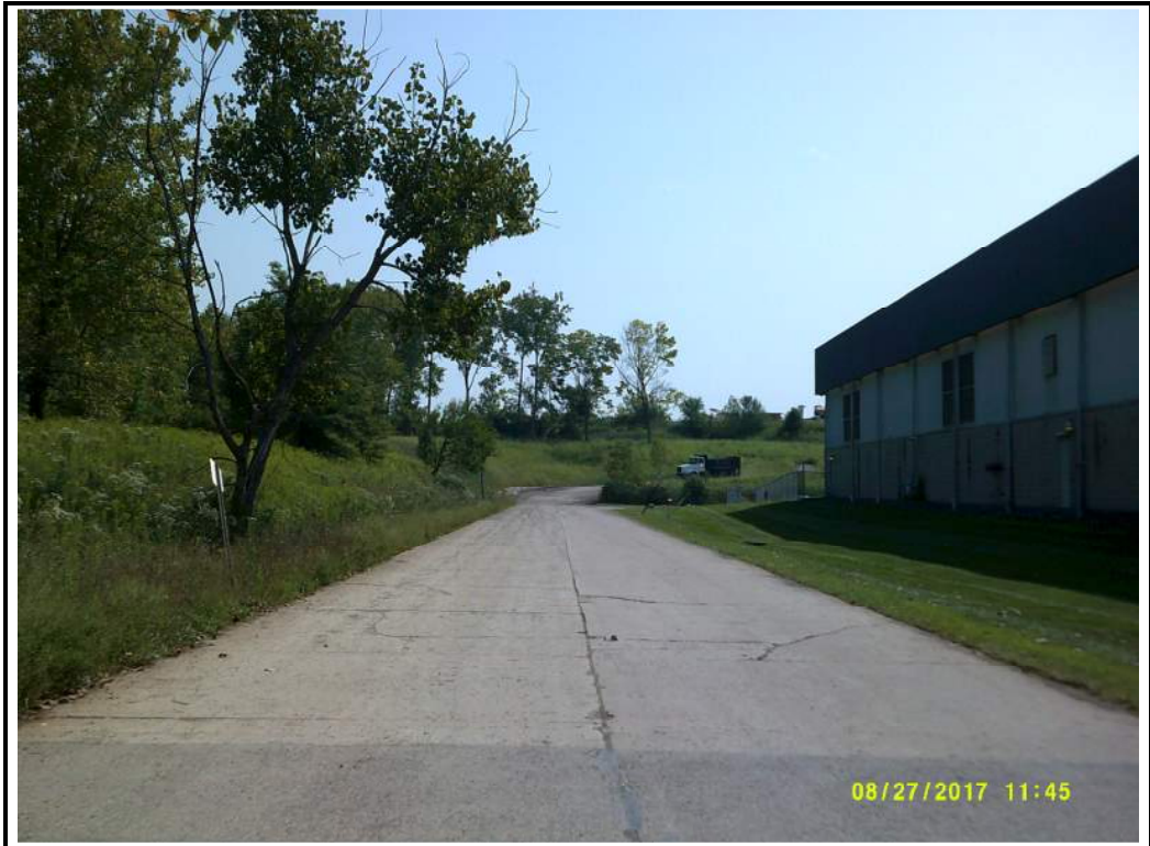
Photograph 27: Leavitt Service Road half way (Arrow on left).
