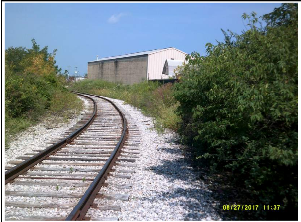
Photograph 15: Rail north toward hedge.
