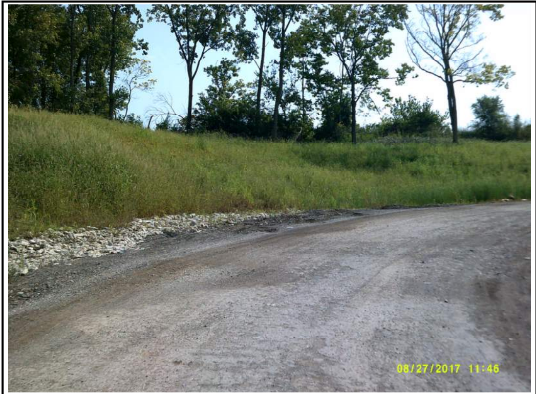
Photograph 29: Geiger Excavating entrance of Leavitt Service Road (looking straight).
