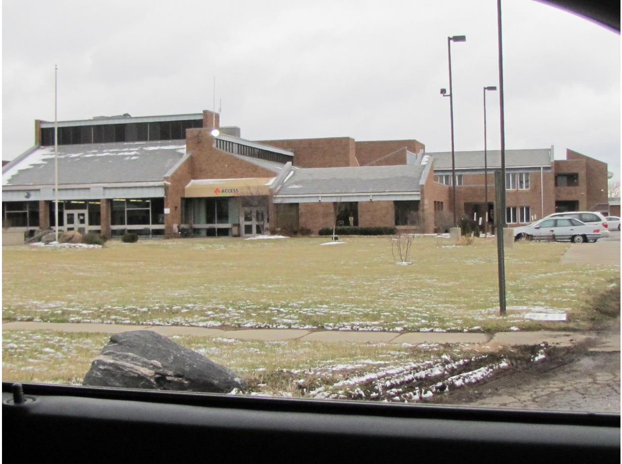
Entrance area at rear of facility.
