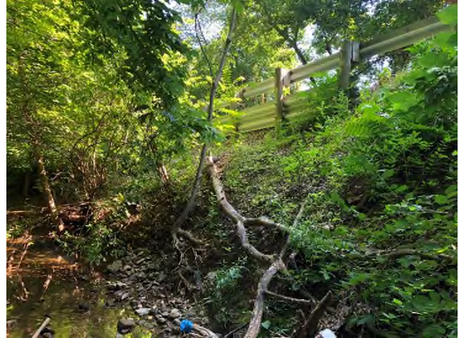
Area 1 Existing Slope – July 15, 2020
