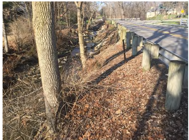
Area 2 Existing Conditions – January 10, 2021
