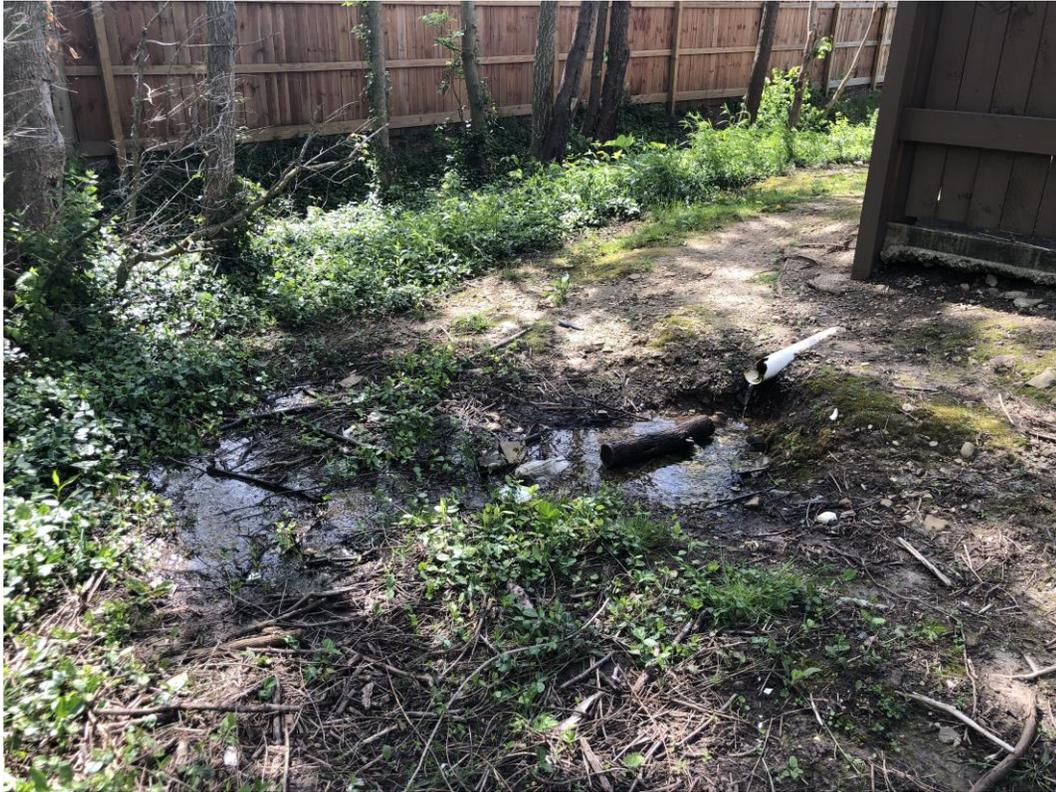
**Photograph 12: Sump pump discharge behind 160 Rocky Creek Drive apartment space**
