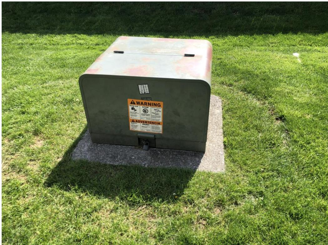
**Photograph 8: One of six pad-mounted transformers along east side of subject property**
