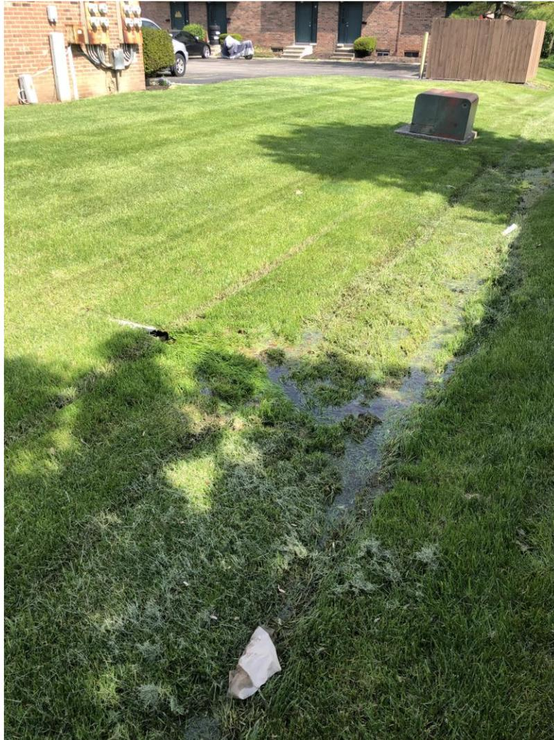
**Photograph 11: Sump pump discharge east of 140-158 Rocky Creek Drive building**
