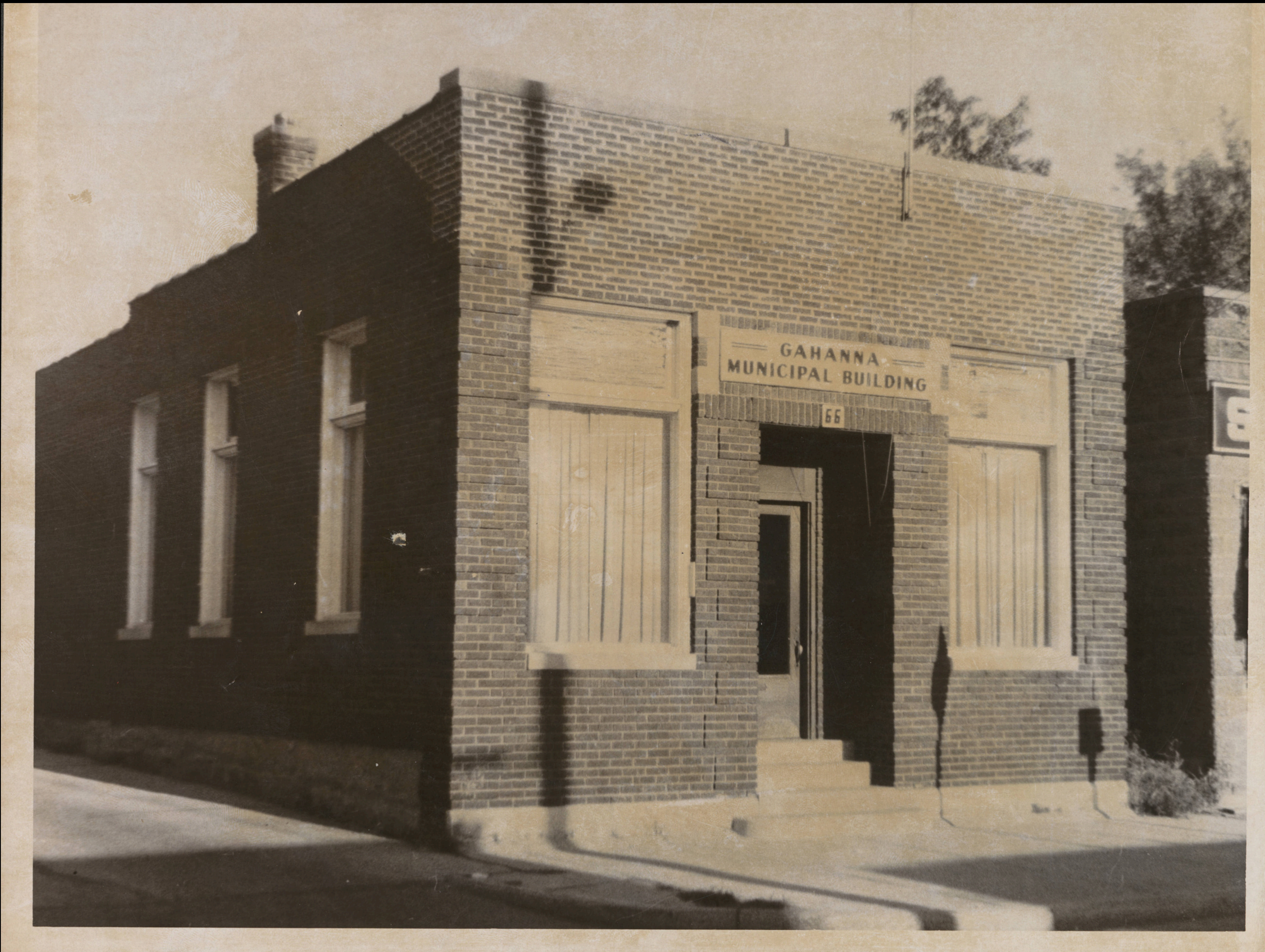
66 S. Mill St. Gahanna Municipal Building, 1959-1979.
