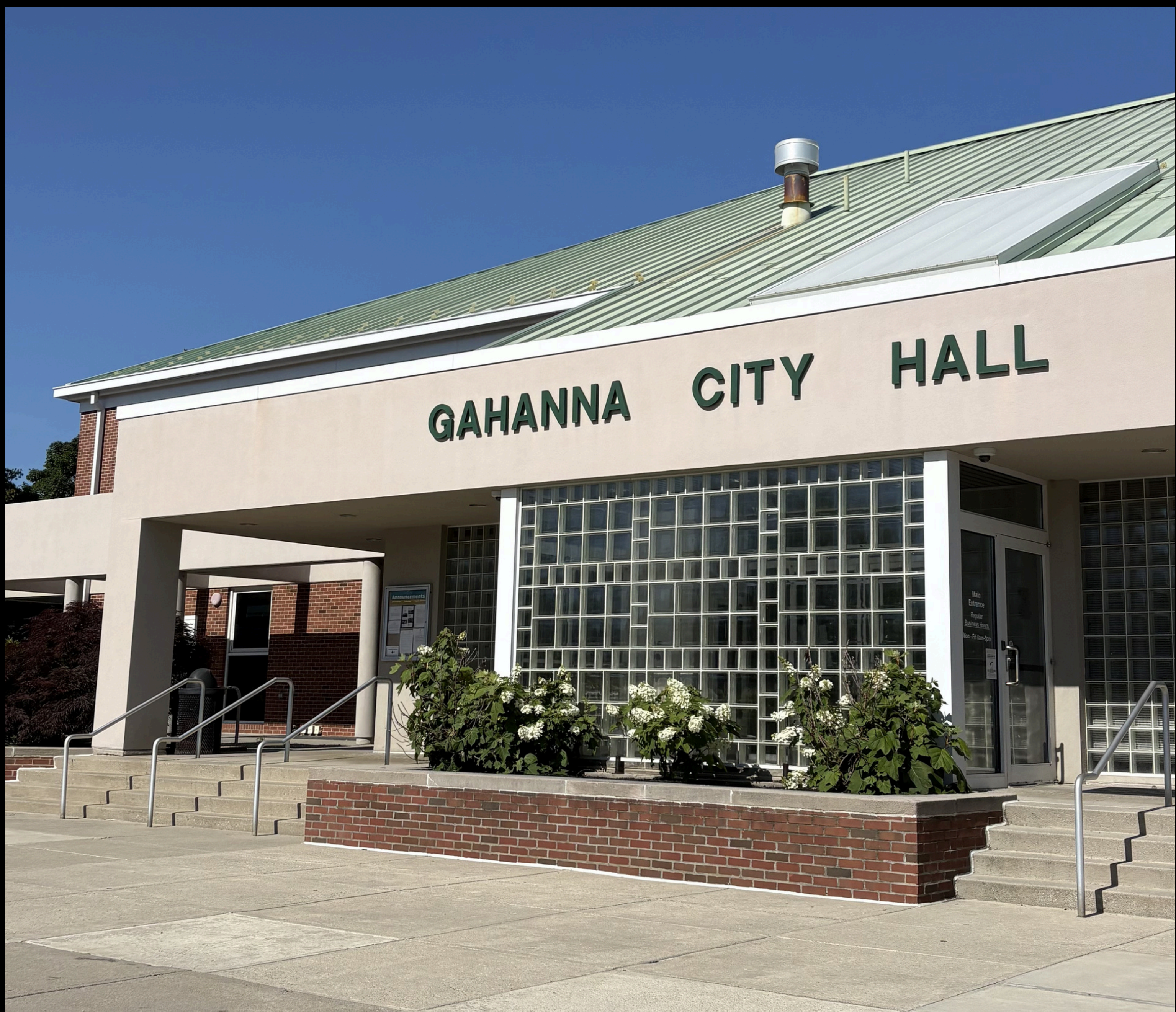
Gahanna City Hall at 200 S. Hamilton Rd., 2020.
