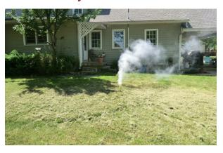
This subdivision was experiencing excessive I/I during heavy rain events that exceeded the existing pump station capabilities and overburdened the sewer system resulting in unnecessary treatment of the I/I. EMH&T performed smoke testing to locate the areas of infiltration and reported the results to Fairfield County staff for review.
