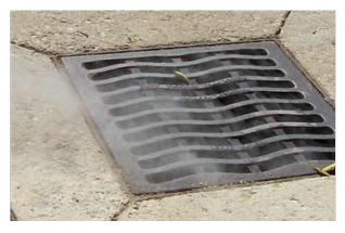
EMH&T's monitoring data and the subsequent analysis collected showed significant amounts of I/I within this portion of the collection system. To further confirm our findings, EMH&T performed an SSES on the area tributary to the Haughn Road sewer. We utilized flow monitoring, smoke testing, manhole inspections, dyed water testing, and closed circuit televising. The study area consisted of approximately 11,300 linear feet of sanitary sewer and 56 manholes.
