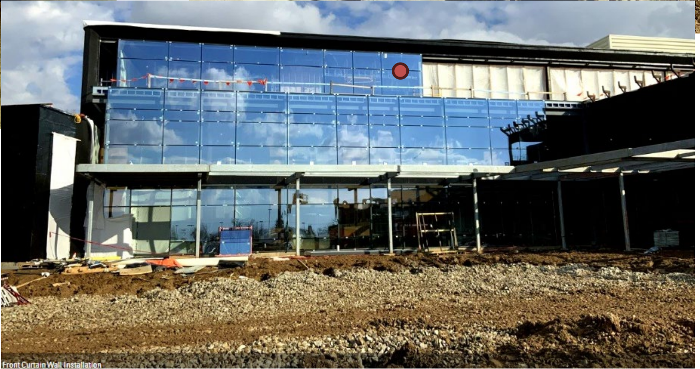
Front Curtain Wall Installation
