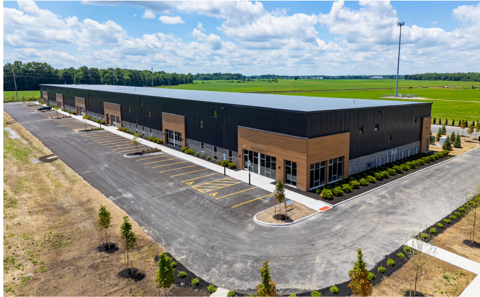
Marysville, OH Completed: 2024
