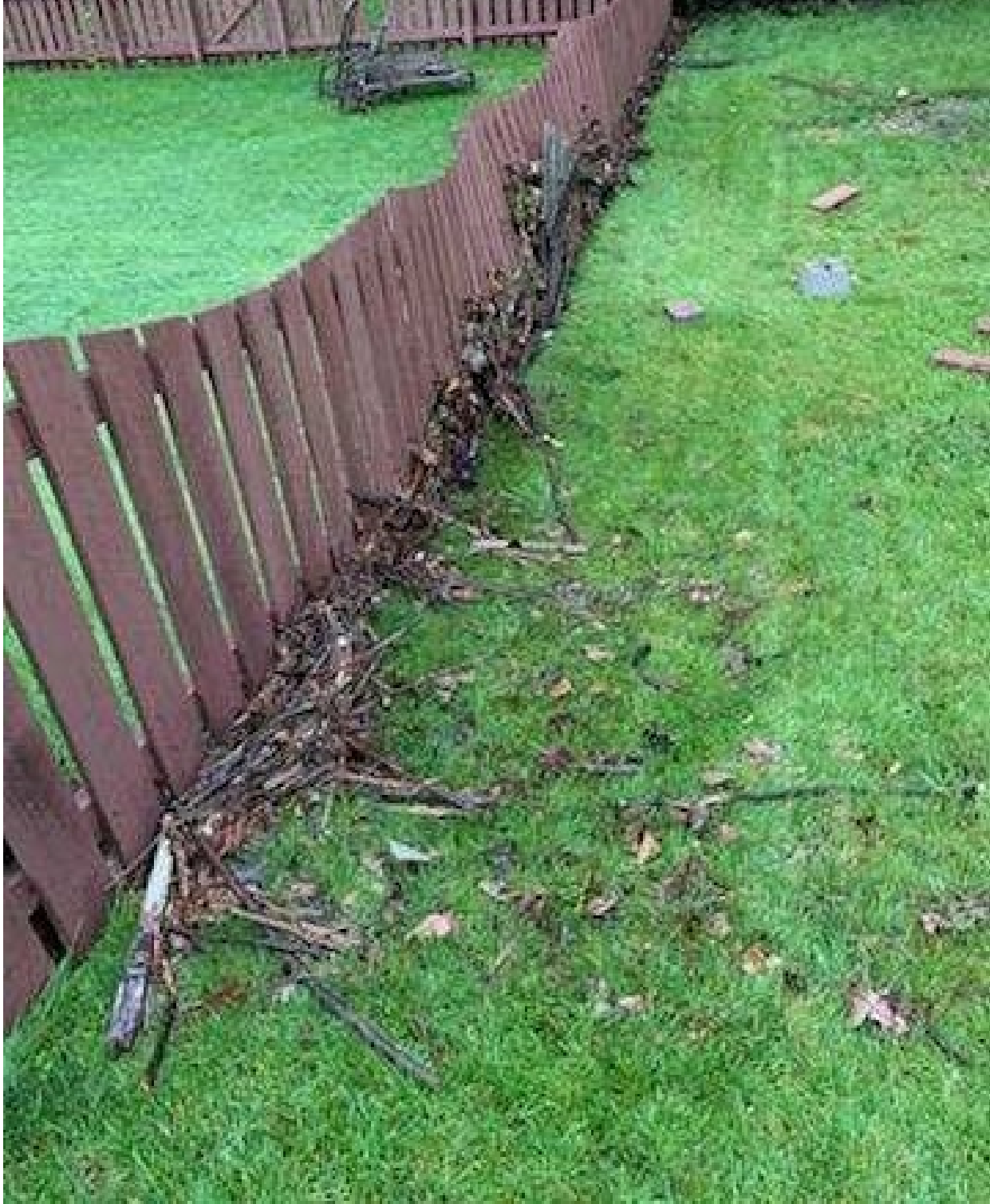
Fig. 6 | June 19, 2019 | Debris collected against the fence on the northwest side of the property. Debris field spanned roughly 30 feet along the fence. The rushing water also damaged the fence by eroding the ground by several of the posts resulting in a weakened fence which tilted >15\% downward. Picture includes one of the other four concrete blocks which supported the bridge. This was moved over 70 feet from my neighbors property. There are also sections of another neighbor's fence which was ripped down and displaced over 150 feet.
