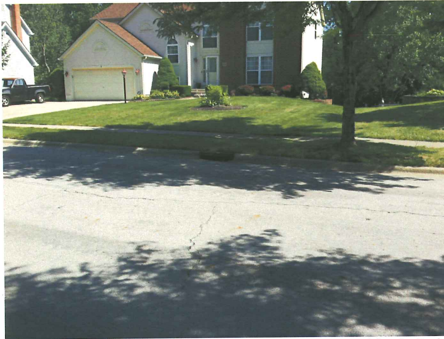
Photograph No. 3 – Facing north across Ashmead Drive toward Souder Ditch
