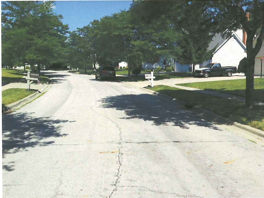
Photograph No. 1 – Ashmead Drive, facing west from the existing catchment basin
