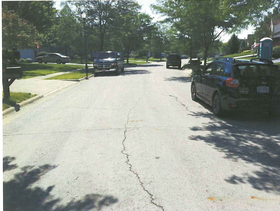
Photograph No. 2 – Ashmead Drive, facing east from the existing catchment basin
