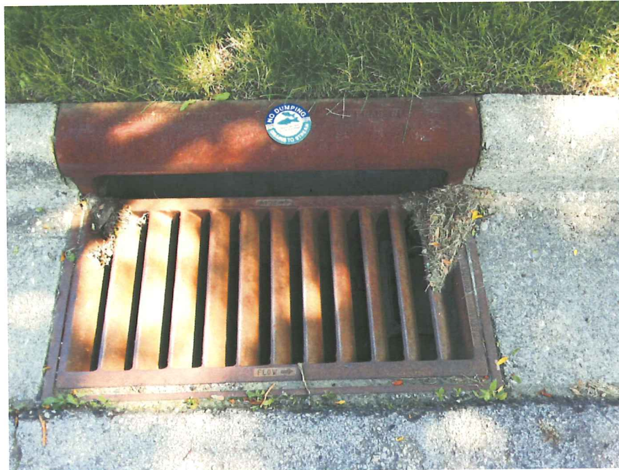
Photograph No. 4 – Existing storm drain on Ashmead Drive
