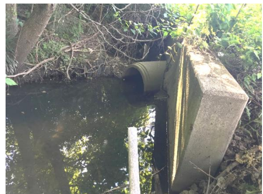
The new waterline will require at least 18” vertical clearance to the existing 18” storm culvert extending under Claycraft Road.
