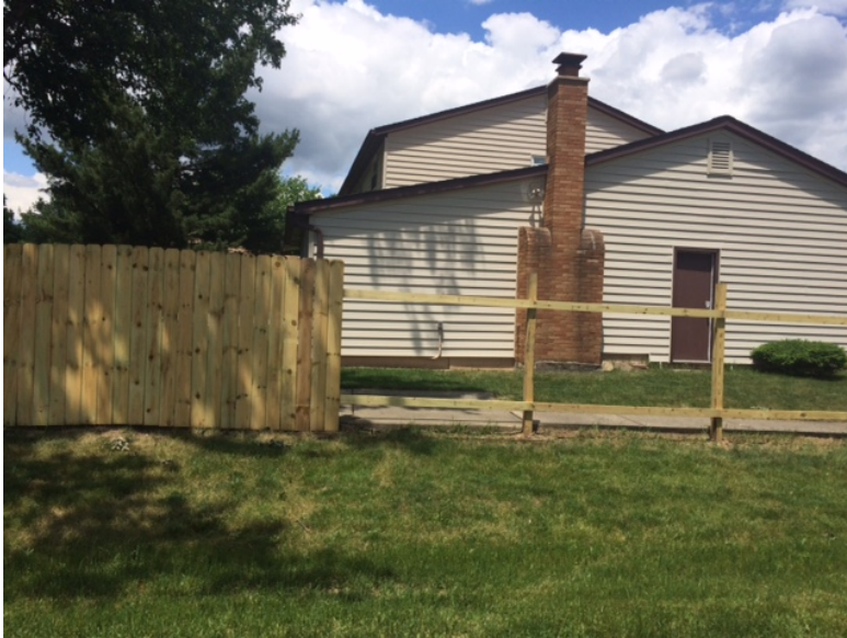
Side yard with fence waiting to be installed.
