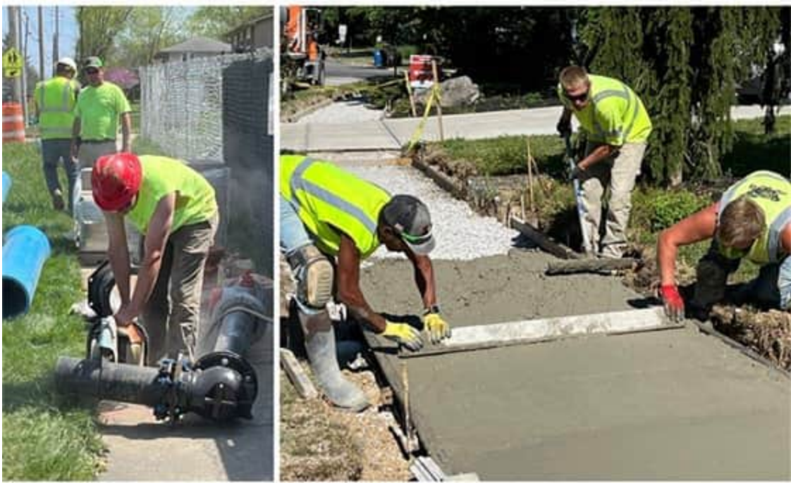
1) Waterline replacement; 2) sidewalk maintenance
