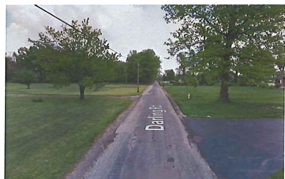
Darling Road B (Looking East)
