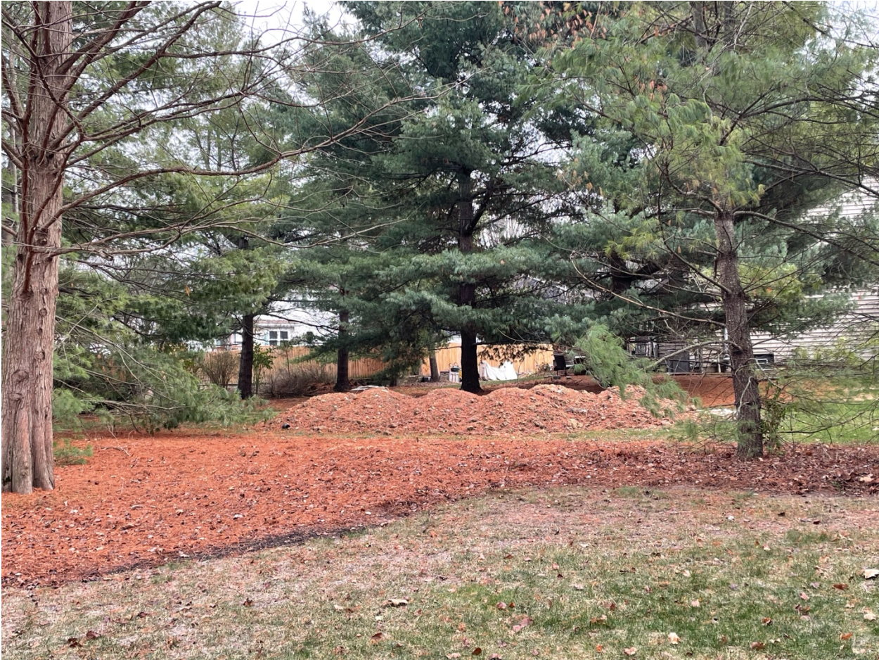
Dirt from excavation done before getting a permit
