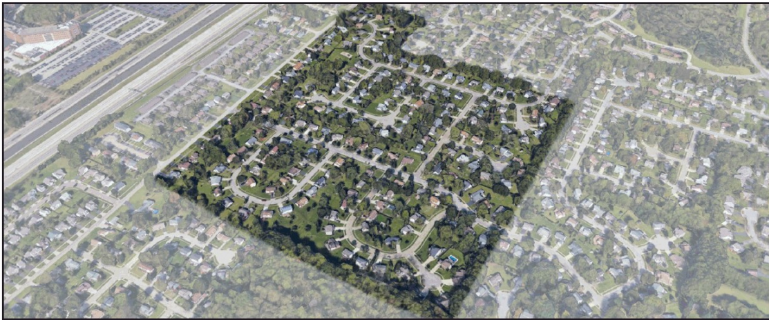
Figure 19: Small Lot Residential includes several distinct geographic areas and may include the area depicted in the image above. For the official zoning map, please visit the City of Gahanna's website.
